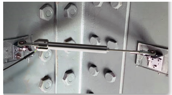
Steel structure monitoring
